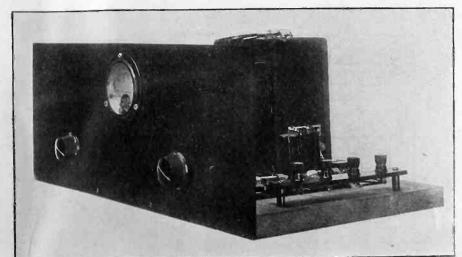
glow tube voltage regulator. When the line voltage goes up, a greater amount of current is by-passed thru the glow tube, thus keeping the 90volt tap constant. In operation, a pink light a p e ars around the elements in the glow tube THE SIMPLEST CONSTRUCTION JOB
